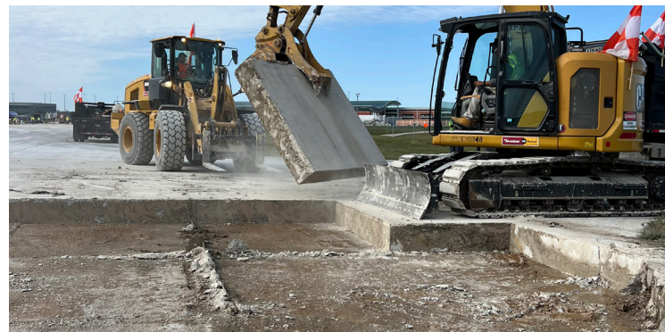
Pavement repairs at the Gerald R. Ford International Airport in Grand Rapids, Michigan, capturing pavement demolitions
